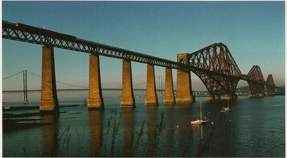
Figure 2.1 The Forth Railway Bridge
